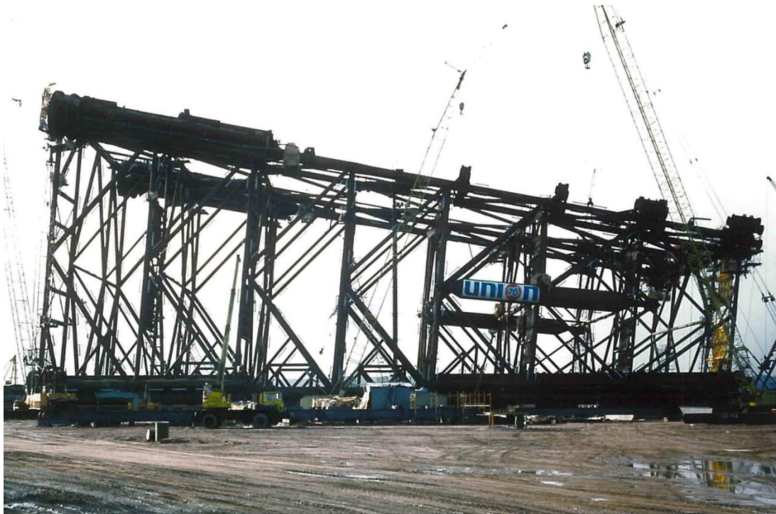
Figure 2.1.2: Heather jacket being fabricated at McDermott Scotland, Ardersier
