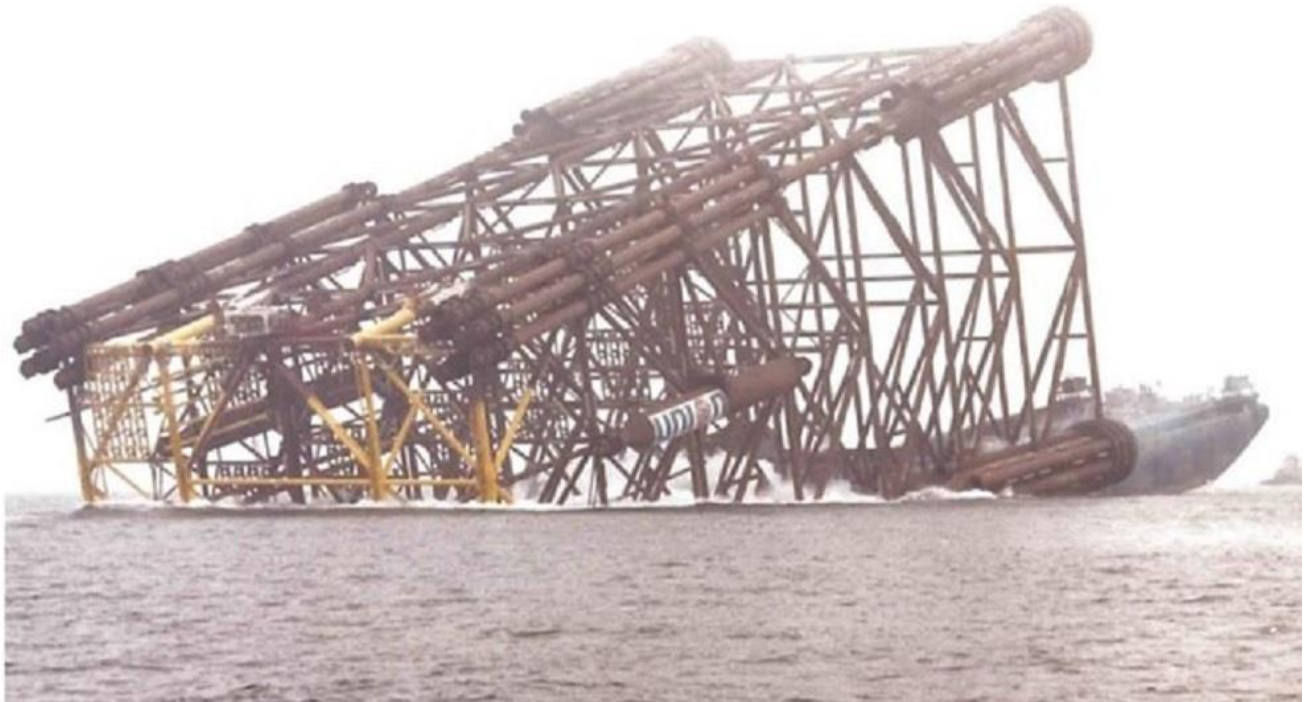
Figure 2.1.3: Heather jacket launch from McDermott Intermac 600
