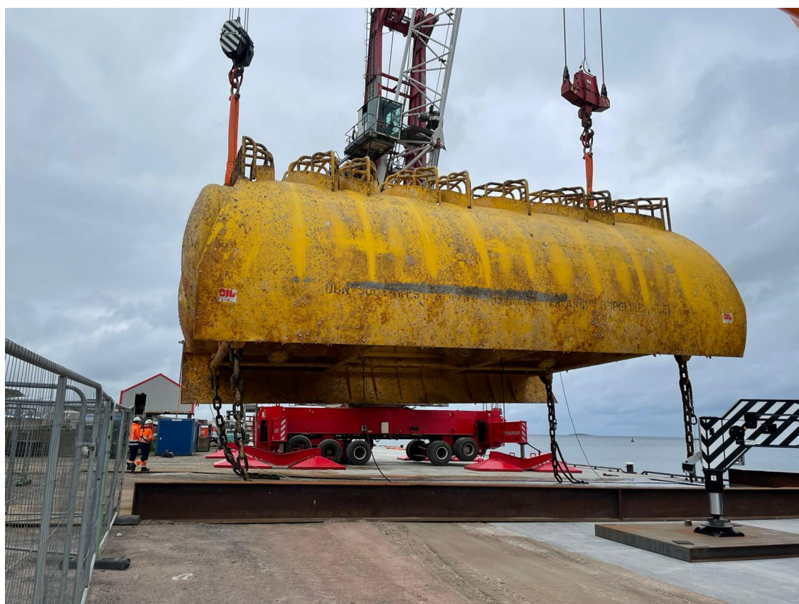
Figure 9.5.4: Mid-Water Arch lifted onto quayside
