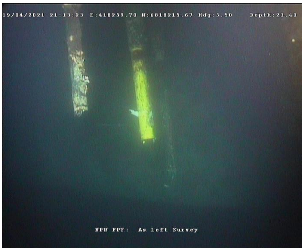
Figure 9.3.2: Cut flexible riser and umbilical
