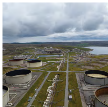
View of Central Avenue Sullom Voe Terminal
