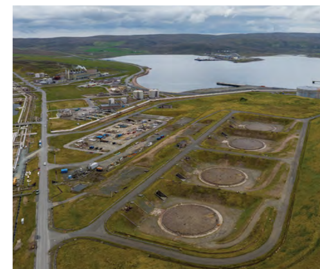
A view across Sullom Voe to the port of Sella Ness showing the four deep-water jetties at SVT
