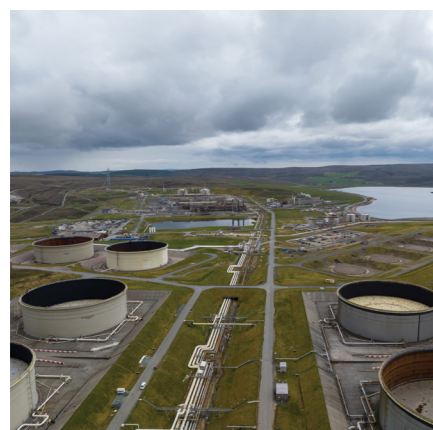
View of Central Avenue Sullom Voe Terminal
