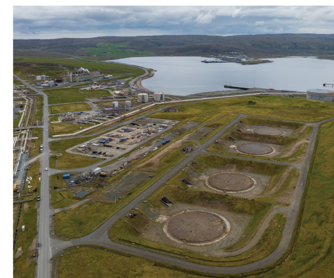
A view across Sullom Voe to the port of Sella Ness showing the four deep-water jetties at SVT
