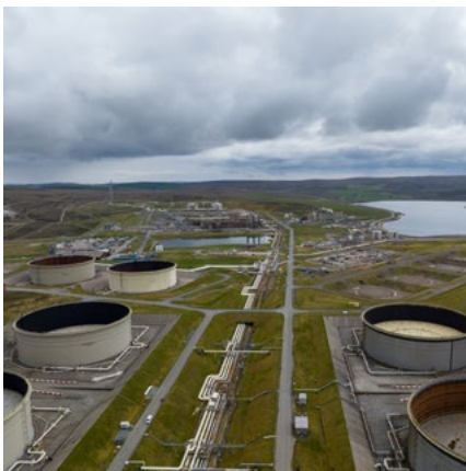
View of Central Avenue Sullom Voe Terminal
